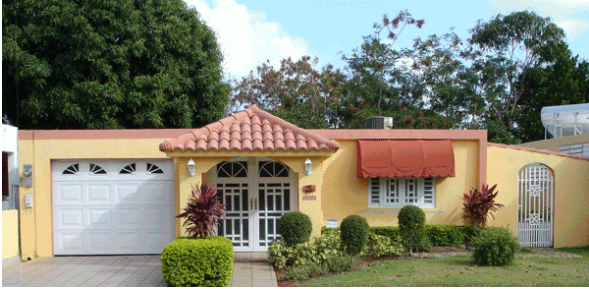
Solar powered & rainwater filtration system.
